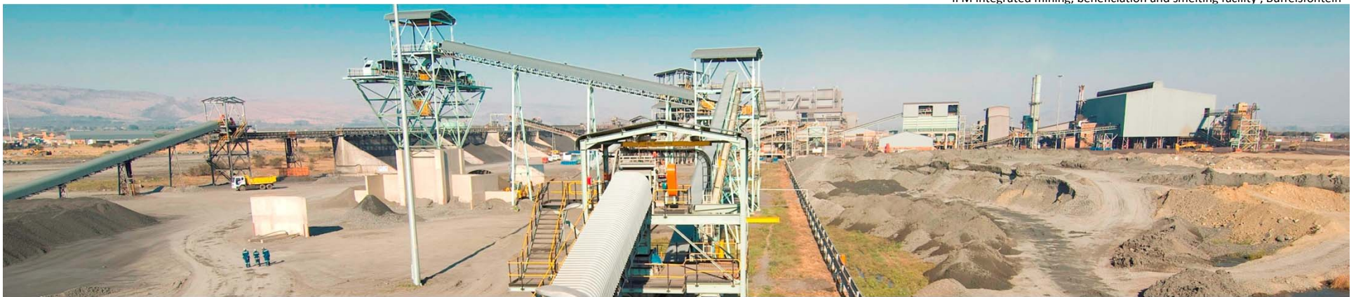
IFM integrated mining, beneficiation and smelting facility , Buffsfontein
